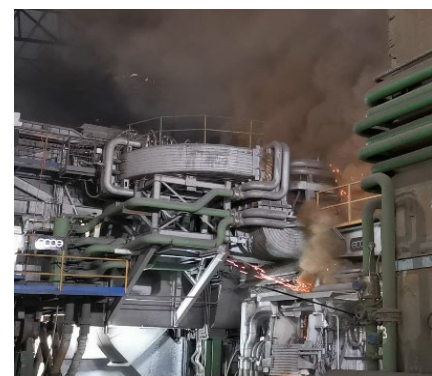
Figure 5 / Cold drilling phase
